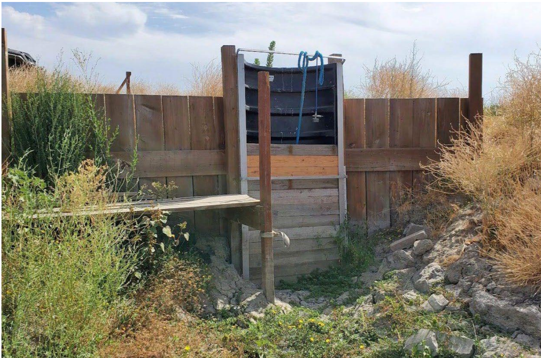
Photo 10. Existing water management structure to allow tide waters onto Bank property (August 5, 2022)
